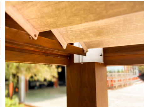
The corner joints are tightened.
