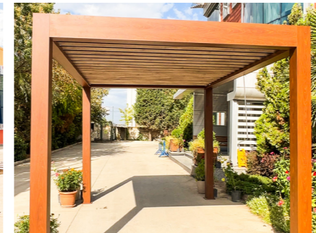
The entire framework assembly is completed.
