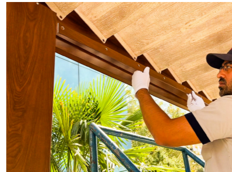
The screw tightening of the panel profiles is completed.
