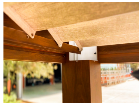
The corner joints are tightened.
