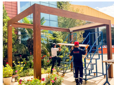
The panel profiles are mounted to the ceiling.
