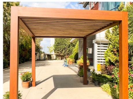
The entire framework assembly is completed.
